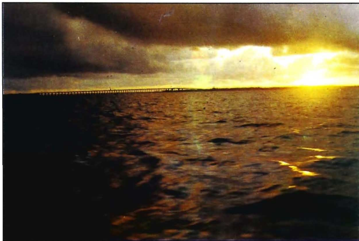
Fig. 1. Indira Gandhi Bridge—The gate way for Gulf of Mannar.
