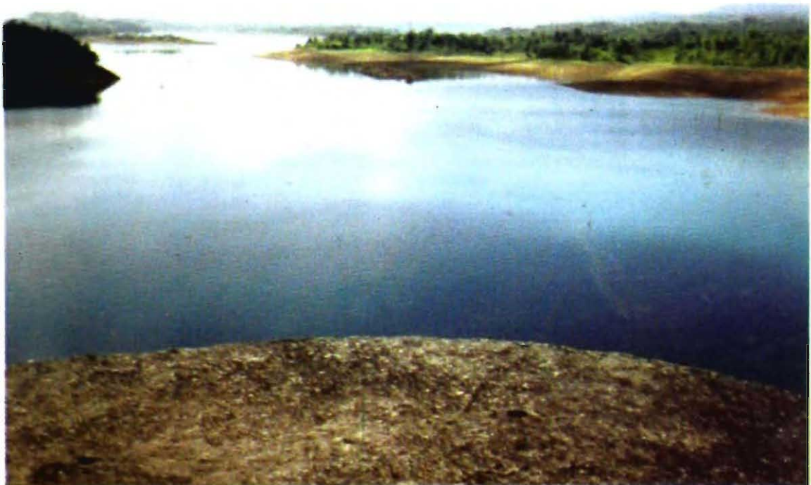
Fig. 6. : View of Umrong reservoir.
