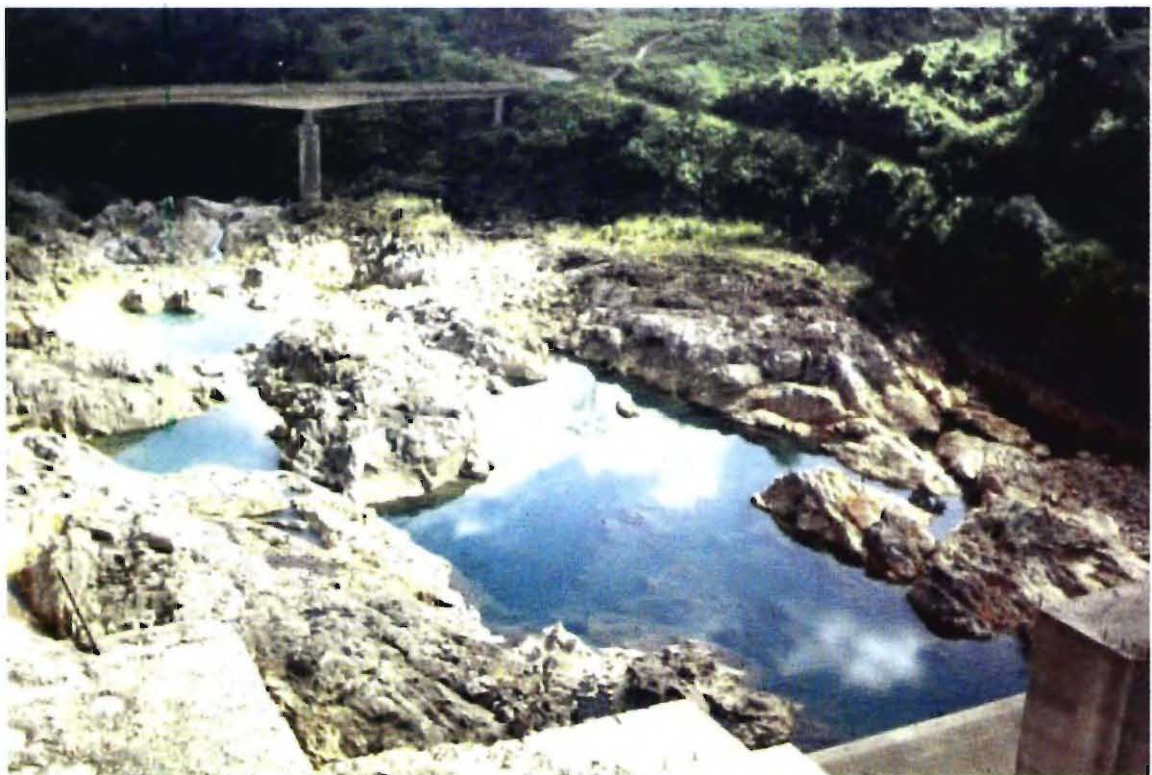
Fig. 2. : Opposite view of Khandong Dam.
