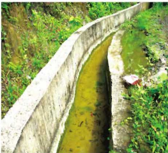
Rain water drainage on Laxmi Nagar
